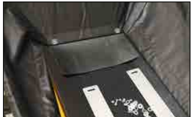
Fig 64 - Tail flashing on top of side flashing
