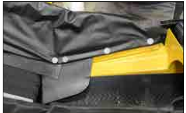
Fig 65 - Transition corner flashing in place
